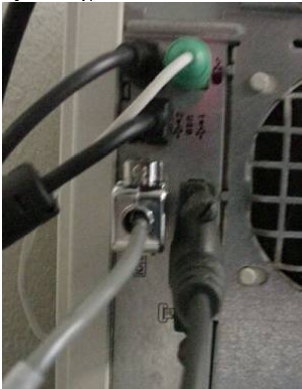
Figure 22. Serial cable connected
